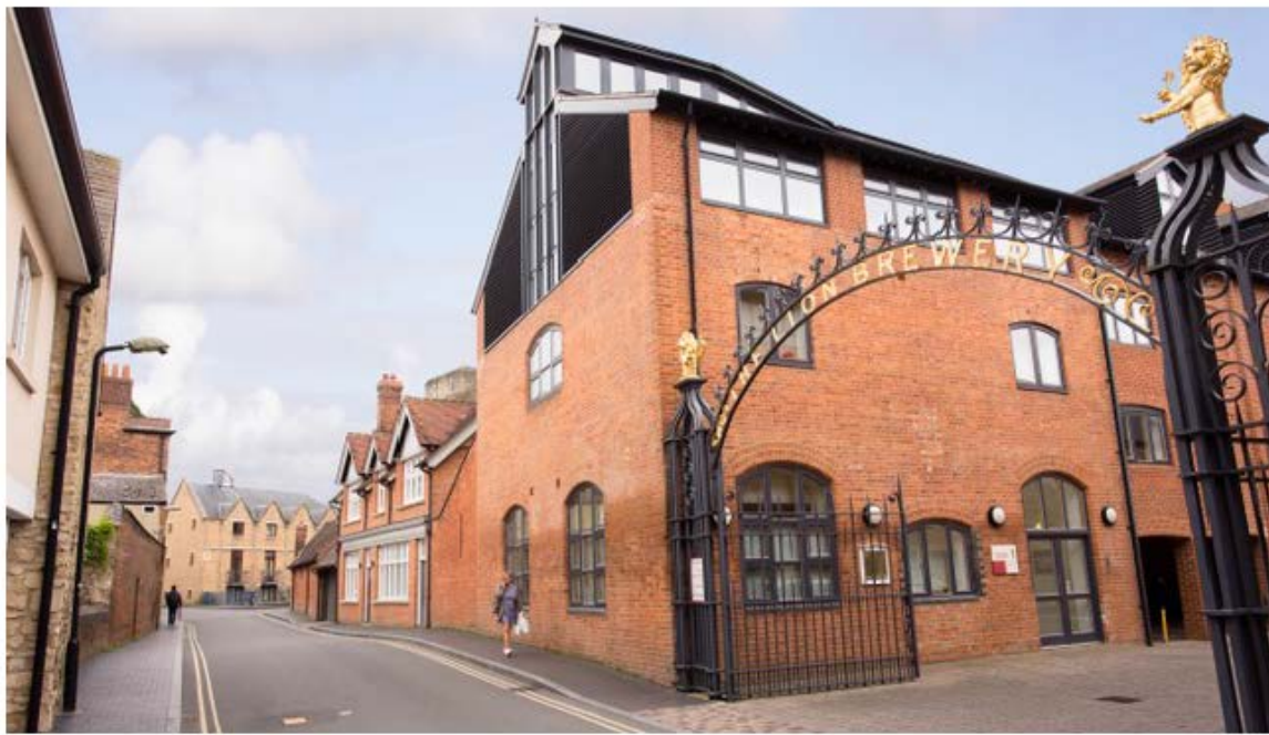
3. Existing view from St Thomas' Street
